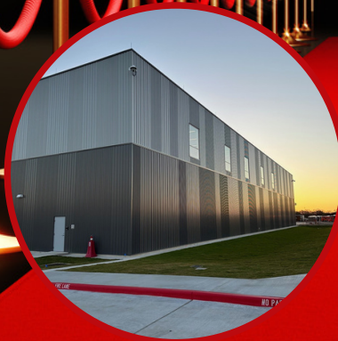
FDBT FujiFilm Building 200 Expansion | Vaughn Construction
