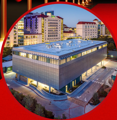
Houston Zoo Admin. Building & Garage O'Donnell/Snider Construction
