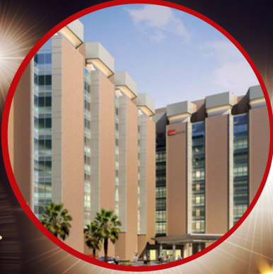
John Sealy Modernization Hensel Phelps
